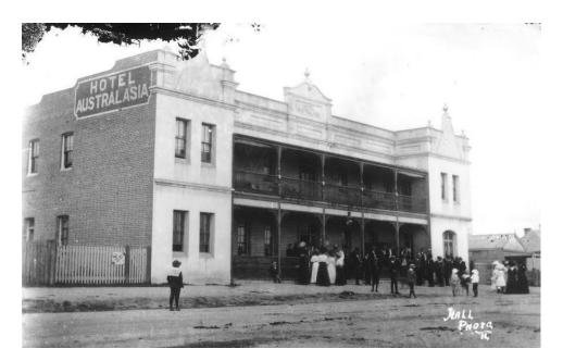
Note the decorative treatments to the upper parapet, and the interesting contrast between the rendering to the front face of the wings compared to the brickwork beneath the verandah.
